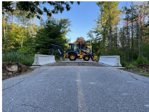
The Fairbanks Street culvert ready for new pavement.
