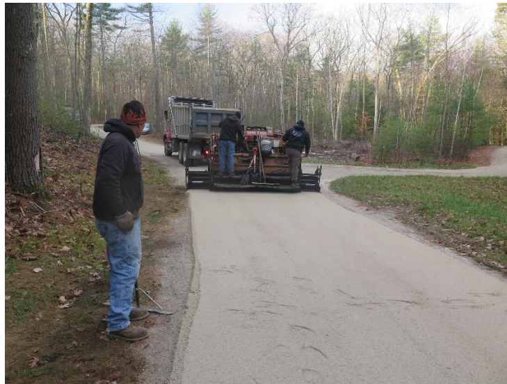
Manning to River stone dust paving
