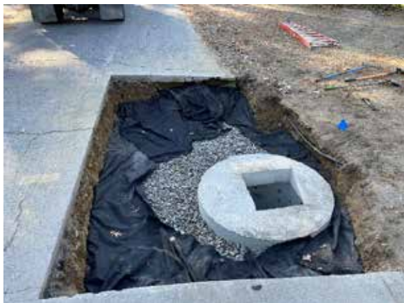
Installing a new catch basin on Clemence Ave
