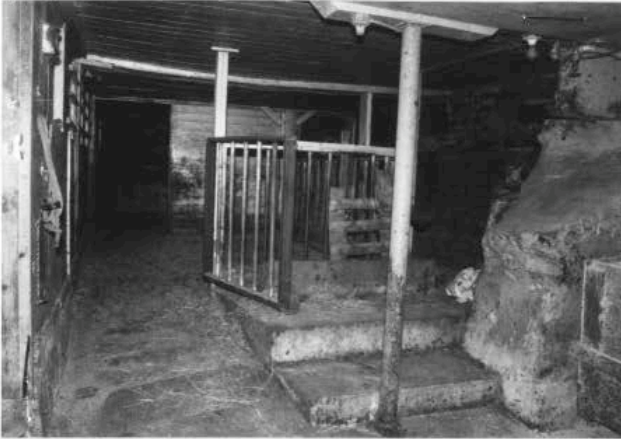
Wagon house, cellar level. 2001.
