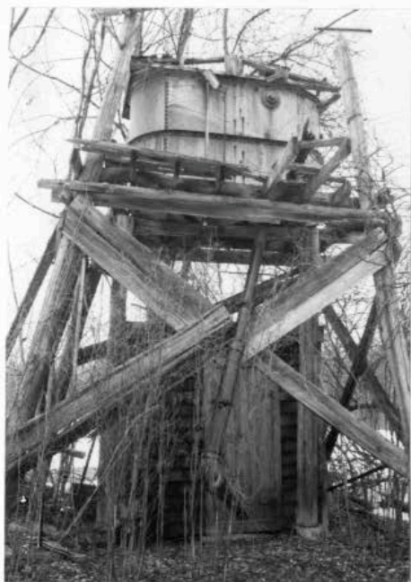
Water tank and pump-house (STE. 954). 2001.
