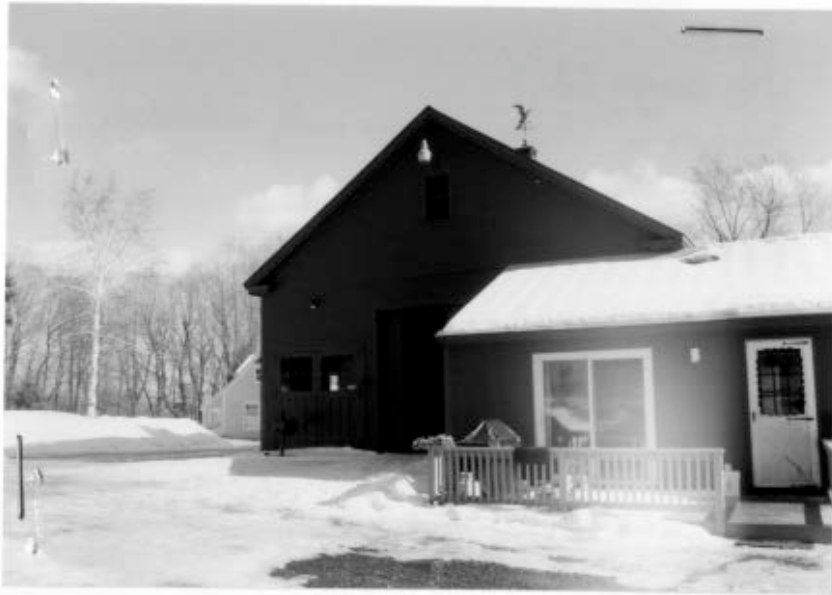
Barn - rear and side wing addition, 2/01.
