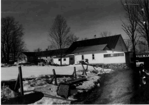
Side of cider house and barn roof, looking NW. 3/01.
