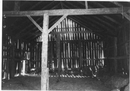
Barn (STE. 416), west wall. 2001.
