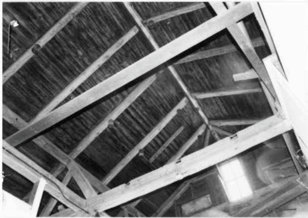
Cow barn - roof. (STE. 516). 2001.
