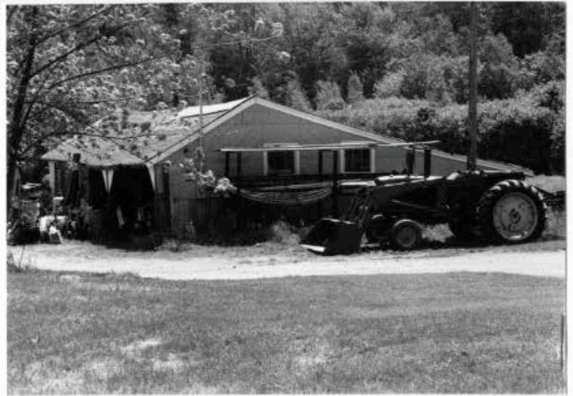
230 Upper North Row Rd - equipment shed. 2001.
