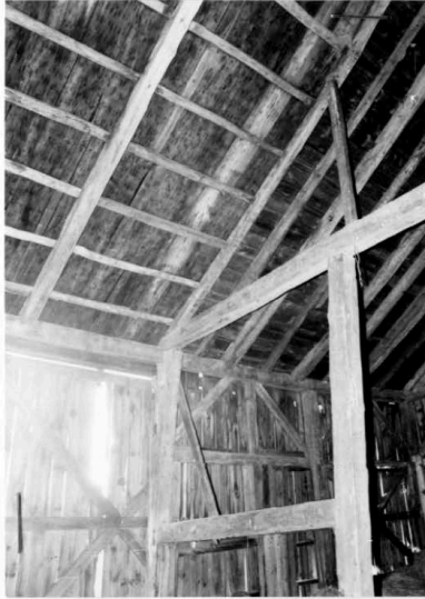
Opposite 132 Redemption Rock Trail - barn (STE. 416), northeast corner view. 2001.
