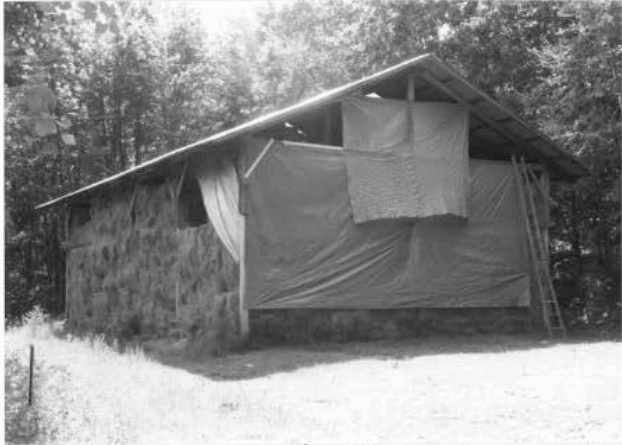
230 Upper North Row Rd - hay barn. 2001.
