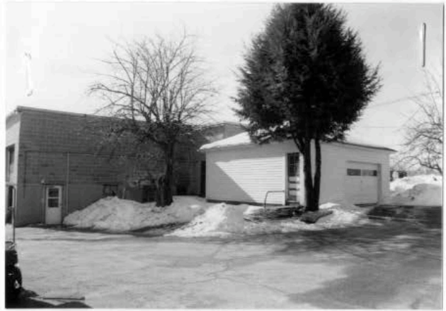
Garage (STE. 375) and apple storage warehouse (STE. 376). 2/01.
