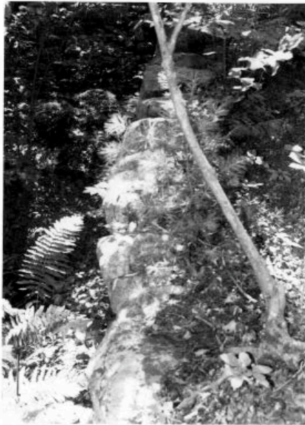
Stuart Sawmill Site (STE.993) Causeway retaining wall. 2001.
