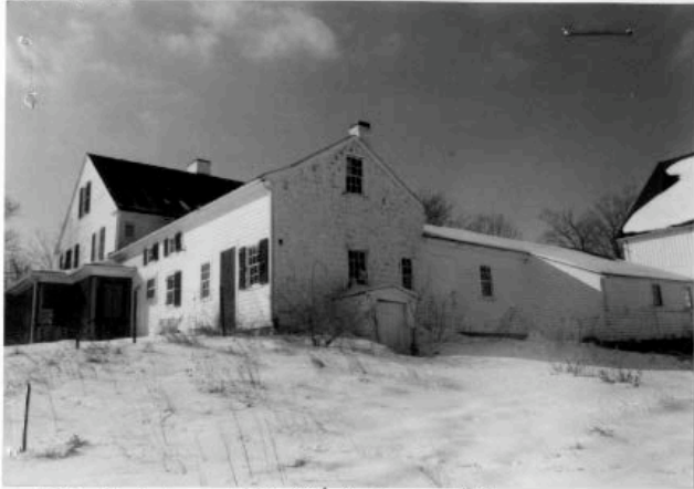
150 Redstone Hill Rd - rear of house, rear ell, and wagon shed. 1/01.
