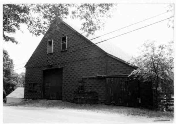
35 North Row Rd - barn. 2001.
