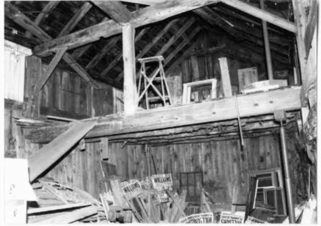
Carriage house interior (STE.340) Facing east. 2001.
