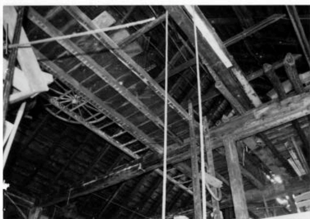
Interior of barn. 5/01.
