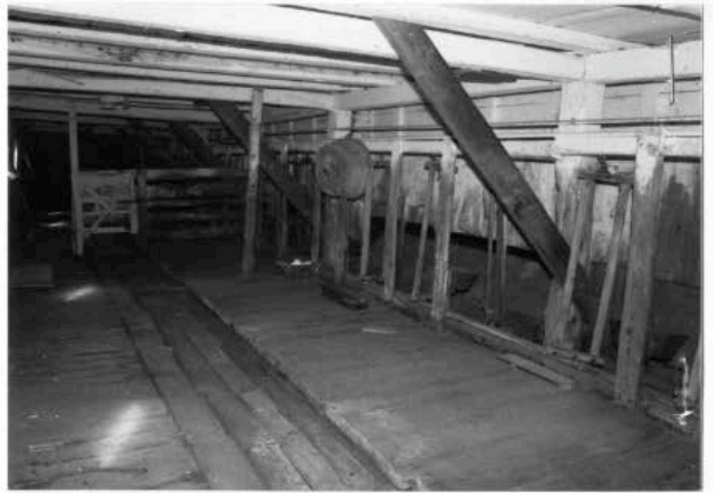
Barn - cow tie-up bay, looking NE. 2000.
