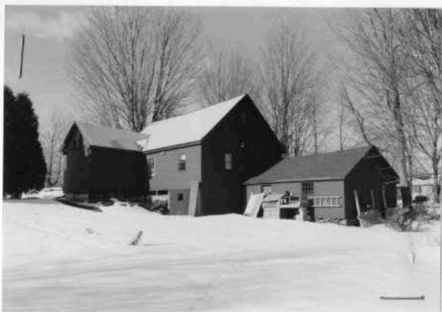
31 Kendall Hill Rd -rear of barn, looking NNW. (STE.367). 2/01.
