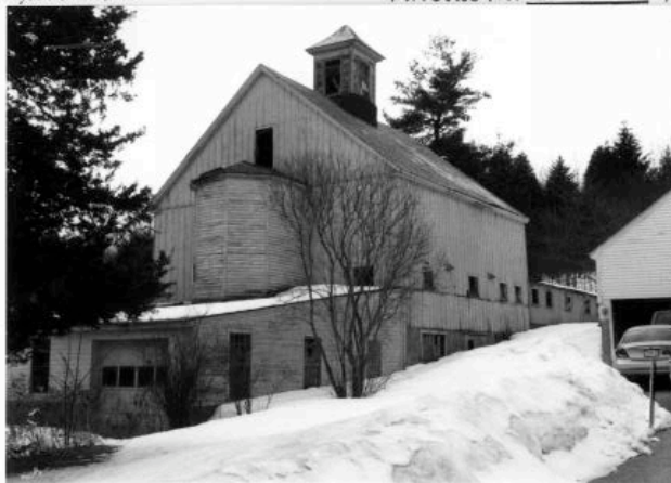
Roper Barn (STE.321) with silo (STE.926) and equipment shed (STE.322). 2001.
