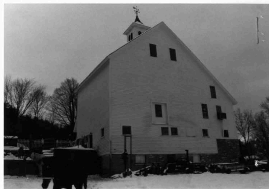
33 Princeton Rd - barn (STE. 406), view south. 2001.
