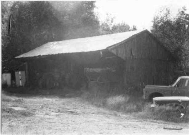
Equipment shed (STE. 537). 2001.
