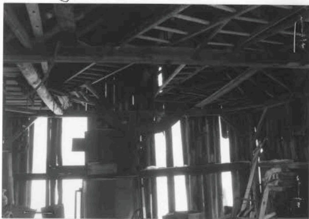
Slaughter house interior and wheel hoist. 1/01.
