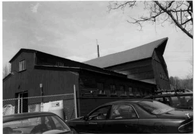
Rear addition to barn. 5/01.
