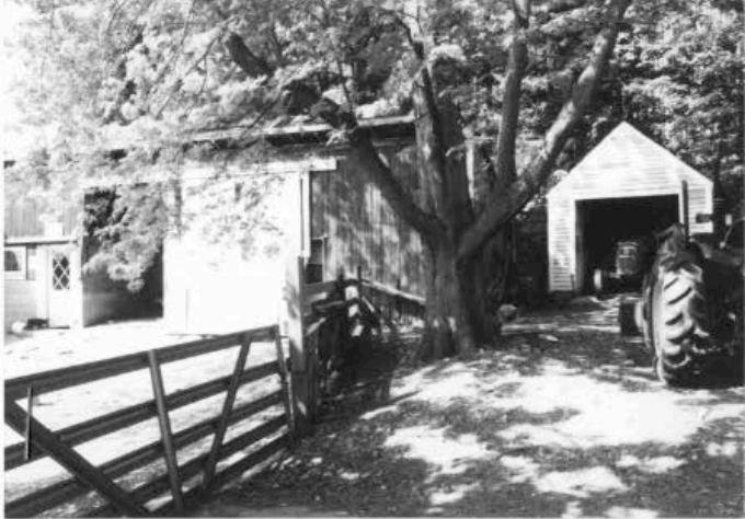
Equipment shed (STE. 458) and garage (STE. 457). 2001.
