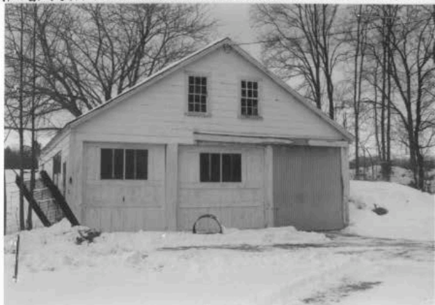
Garage - equipment + shed. (STE. 391). 1/01.
