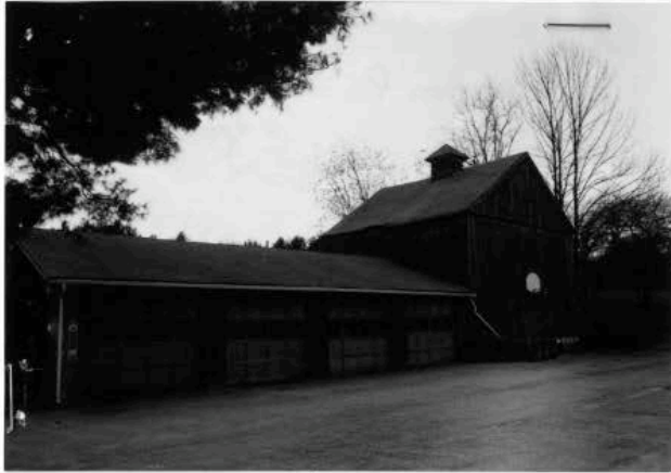
125 Clinton Rd - front of barn and garage wing (STE. 397). 5/01.
