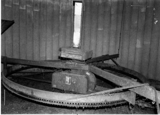
Opposite 132 Redemption Rock Tr. - Silo mechanism (STE. 940). 2001.
