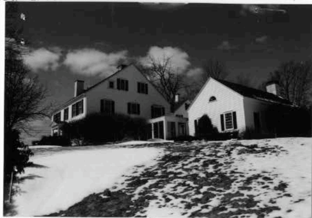
206 Chace Hill Rd - Main house with attached library (STE. 45). 3/01.
