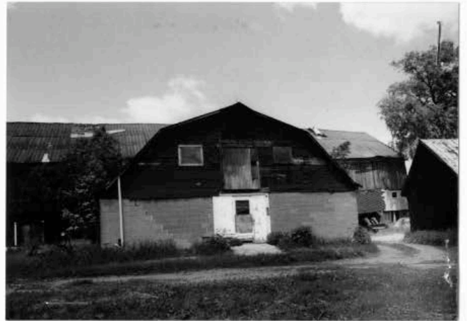
Dairy barn addition (STE. 443). 5/01.
