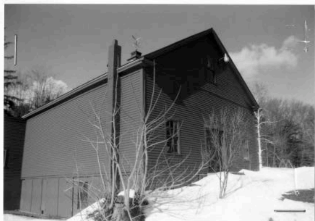
Barn - main facade and south side. 2/01.
