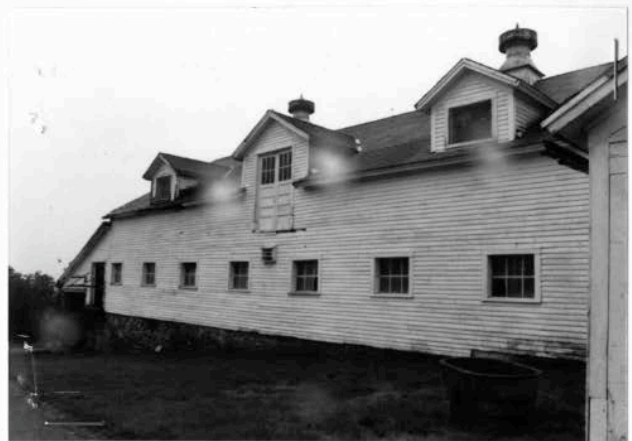
Dairy barn, view SE. (STE. 518). 2001.
