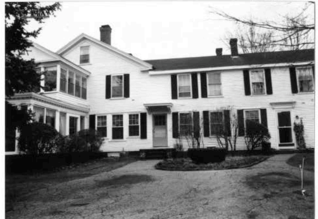
House-gable end, enclosed porches, rear ell 11/00
