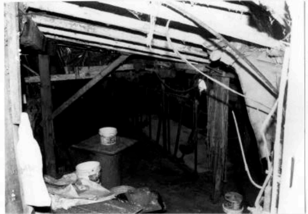
Cow shed (STE. 533), view west.
