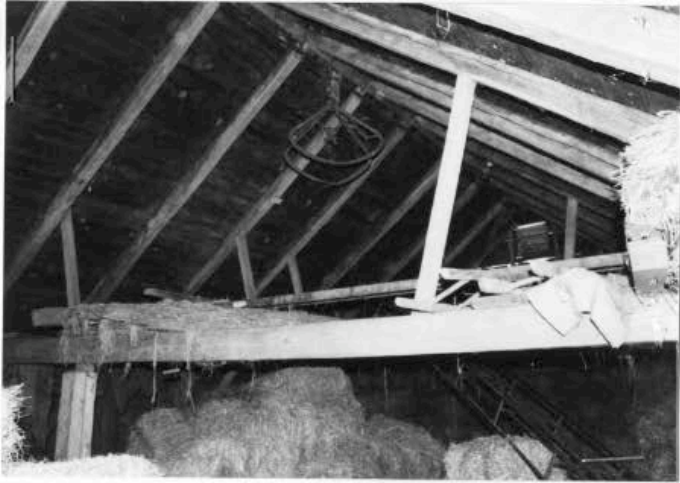
Northeast barn interior, looking east. 2001.
