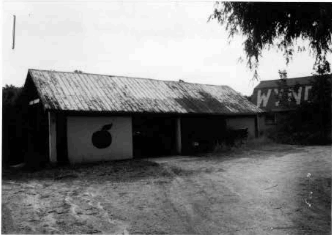
Equipment shed (STE.445). 5/01.
