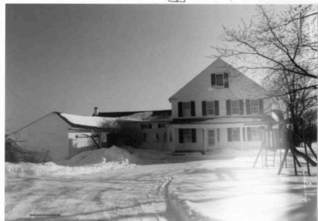
150 Redstone Hill Rd - West side of house and wagon shed (STE. 578). 1/01.
