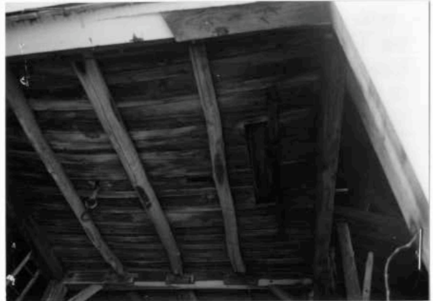
Barn-center scaffold w/wheel for hay hoisting. 5/01.
