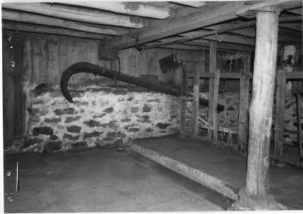
Interior of barn cellar. 2000.
