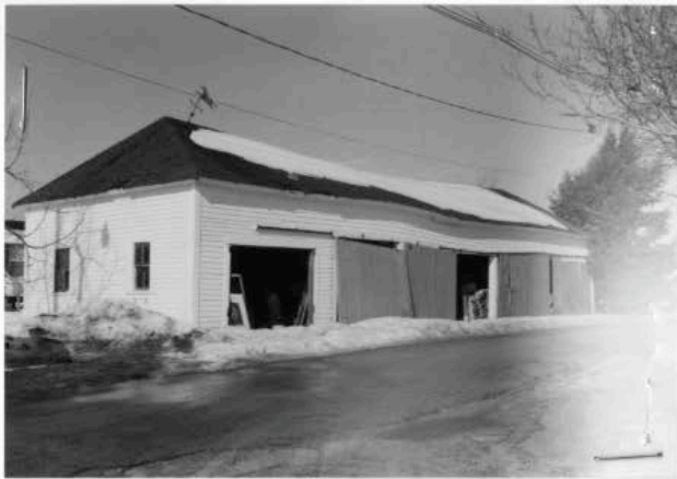
Equipment shed (STE. 374). 2/01.
