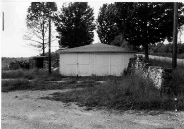
Opposite 43 North Row Rd - root cellar (STE. 975) and garage (STE. 488). 2001.
