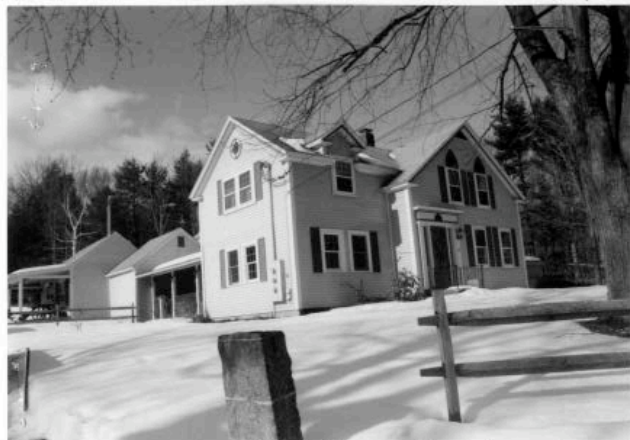
House - south side and main facade. 2/01.
