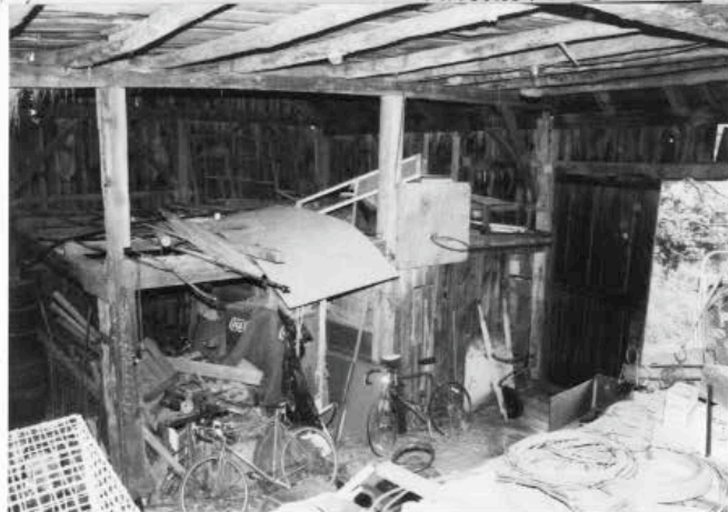
Barn, view southeast. 2001.
