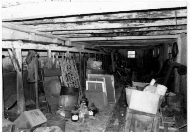
Barn, east aisle (cow-tie aisle) facing N. 2001.
