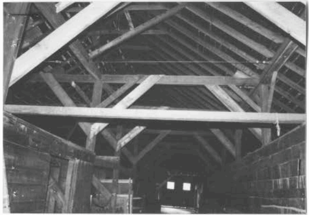
Barn - center aisle looking south. 2000.
