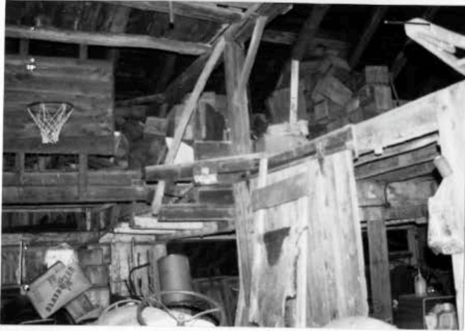
Barn - SE view, "showing cut-off loft joists." 2001.
