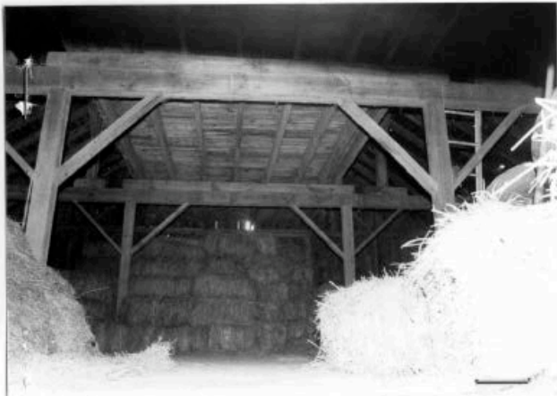
Barn - view north to rear addition - upper level (STE. 532). 2001.
