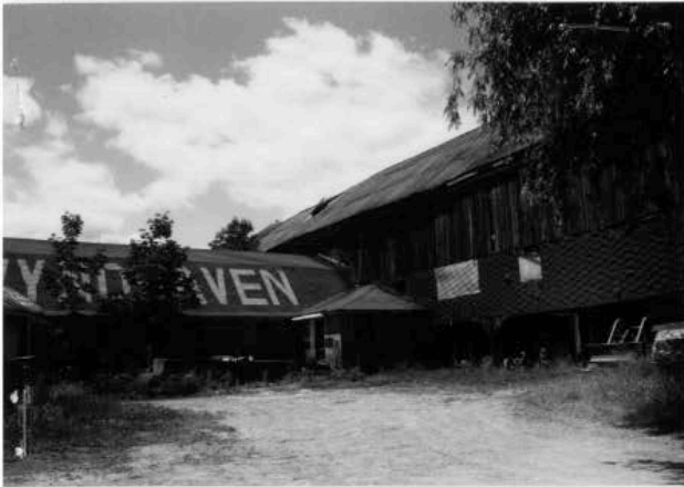
Dairy barn addition (STE.443). 5/01.
