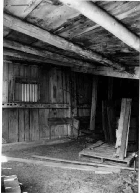
Interior-small barn/wagon shed/ poultry barn (STE.444). 5/01.
