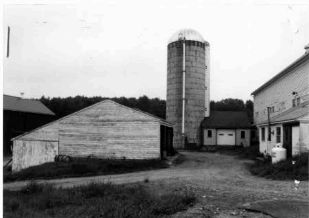
Equipment shed (STE.467), silo/shed (STE.964) and milk room (STE.466). 2001.
