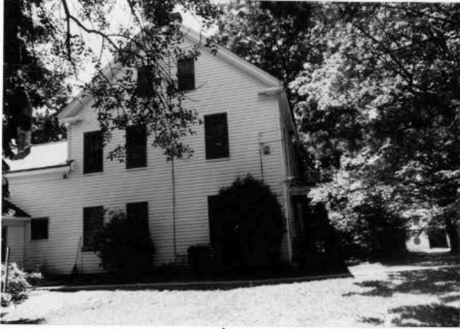
House - side elevation, looking west. 5/01.
