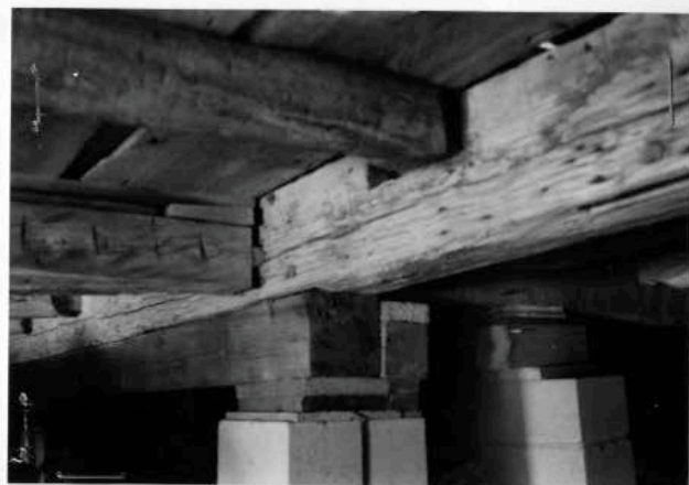
31 Kendall Hill Rd -barn interior -cellar. 3/01.
