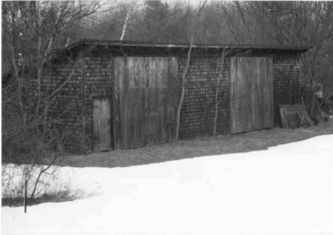
Equipment shed (STE. 455). 2001.
