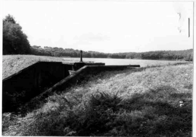
Pond and dam. 2001.
