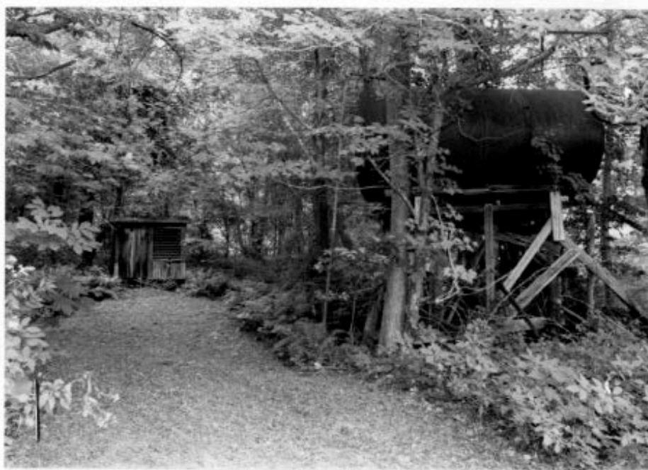
Well/pumphouse (STE. 957) and water tank (STE. 958). 2001.
