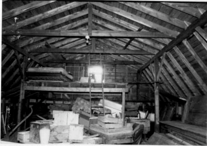
Wilder Heifer barn (STE.324) roof Structure. 2001.
