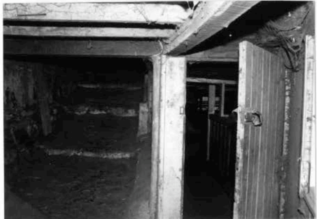
Wagon house, cellar level, cattle ramp (STE. 965). 2001.
