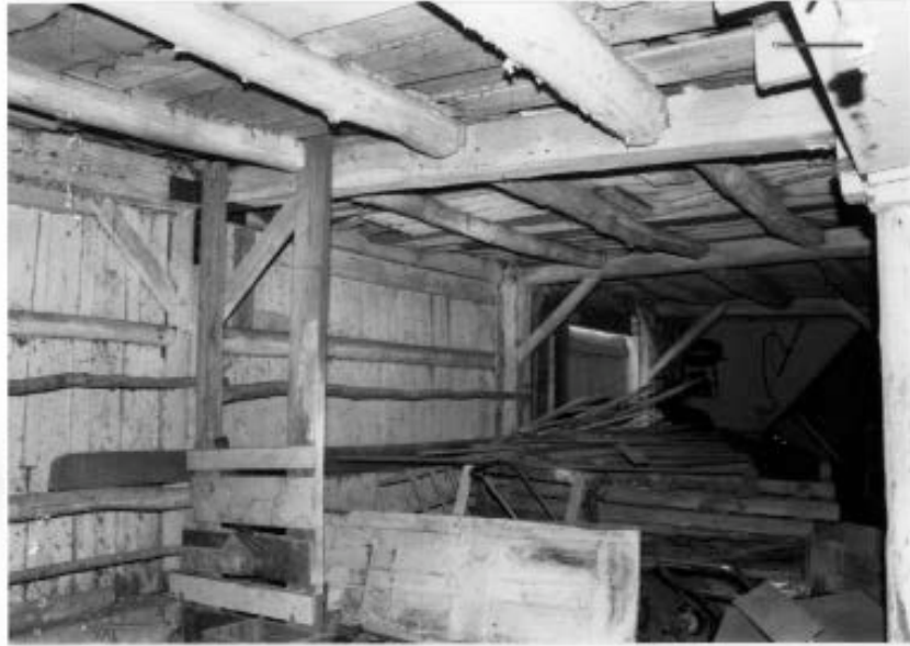
Barn cellar - looking NE. 2001.
