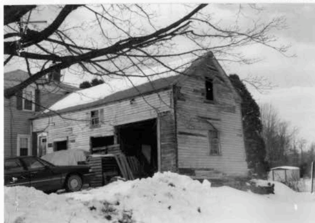
176 Redstone Hill Rd-attached wagon shed. 1/01.
