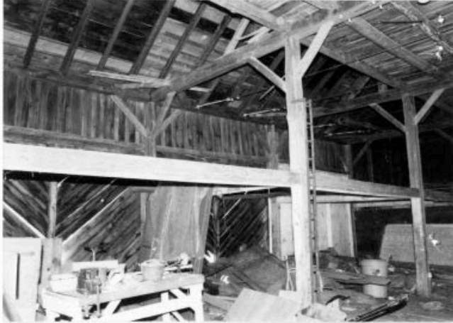
Barn interior. 2001. Facing SW.
