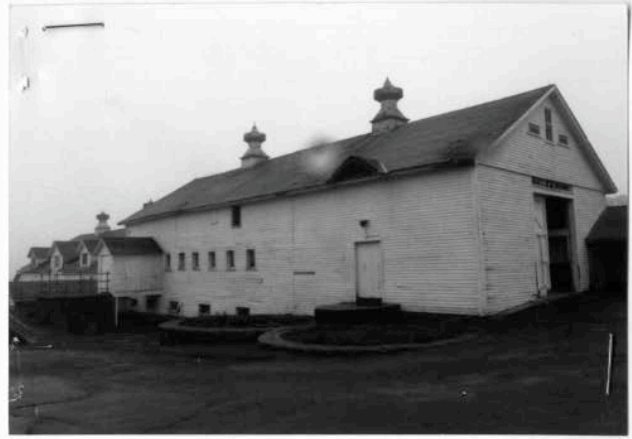
Dairy barn (STE. 518) and cow barn (STE. 516) 2001.
