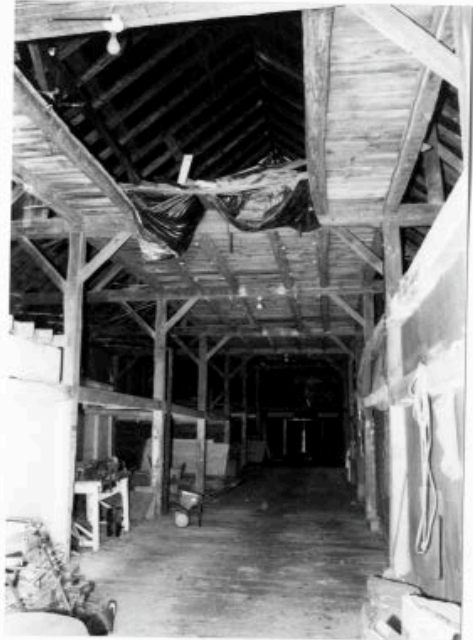
Center aisle of barn, facing west. 2001.
