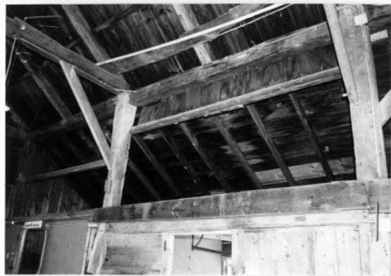
Barn-door header, S. Side. 2001.
