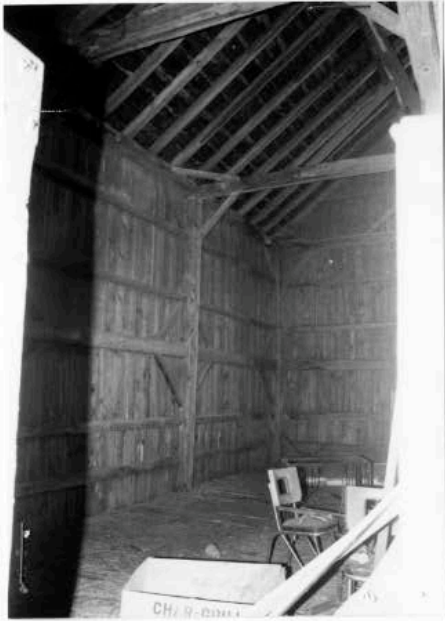
Barn, west aisle facing NW. 2001.
