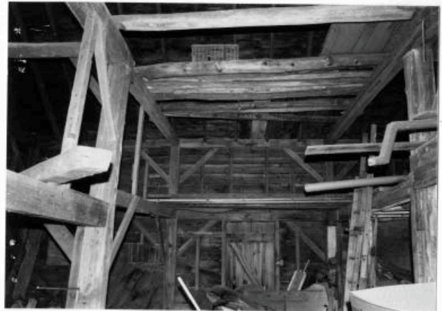
Barn-North in center bay to rear wall. 2001.
