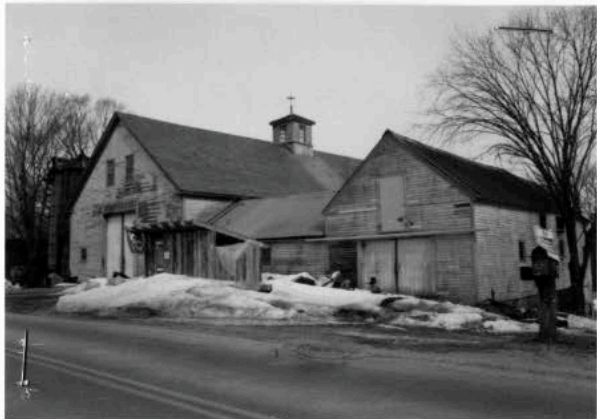
Silo, barn, farmstand, and barn/slaughterhouse. 2001.
