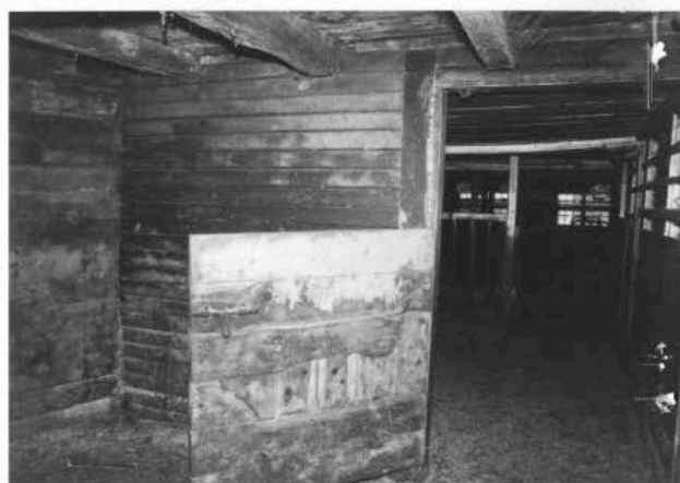
Wagon house, cellar level. 2001.
