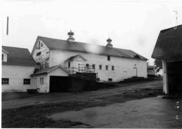
Dairy barn (STE. 518) and cow barn (STE. 516). 2001.
