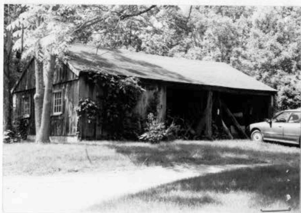
Equipment shed (STE. 491). 2001.
