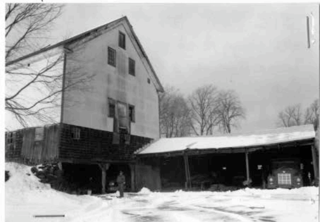
Rear elevation of barn and loading barn (STE. 387 and STE. 389). 1/01.
