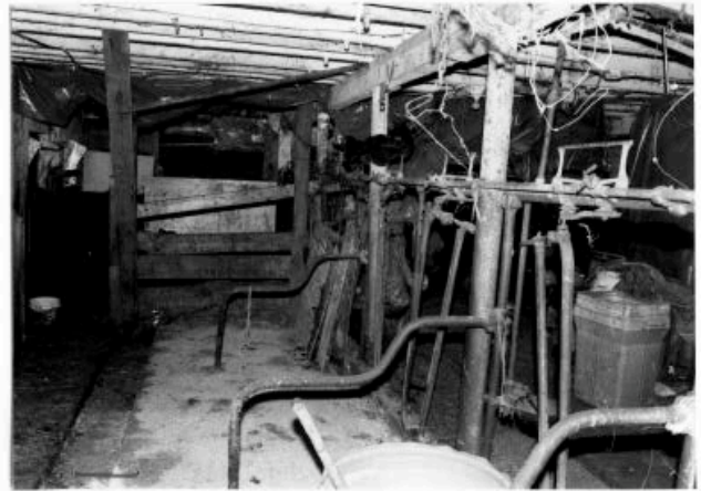
Barn extension - ground floor. 2001.
