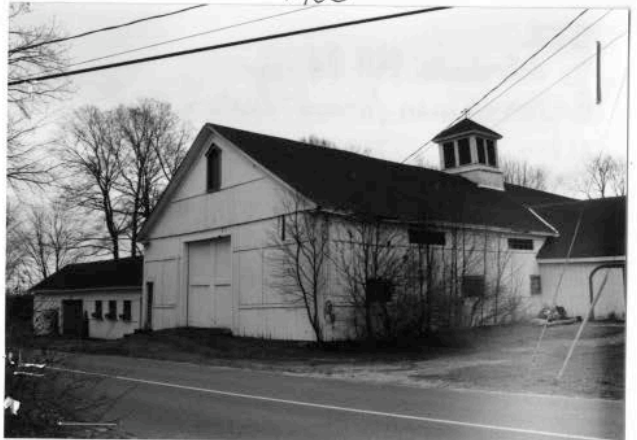
Barn -Main facade looking south. 11/00.
