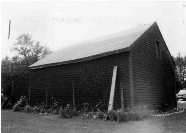
Barn - rear elevation. 5/01.
