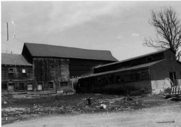
Rear of barn. 5/01.
