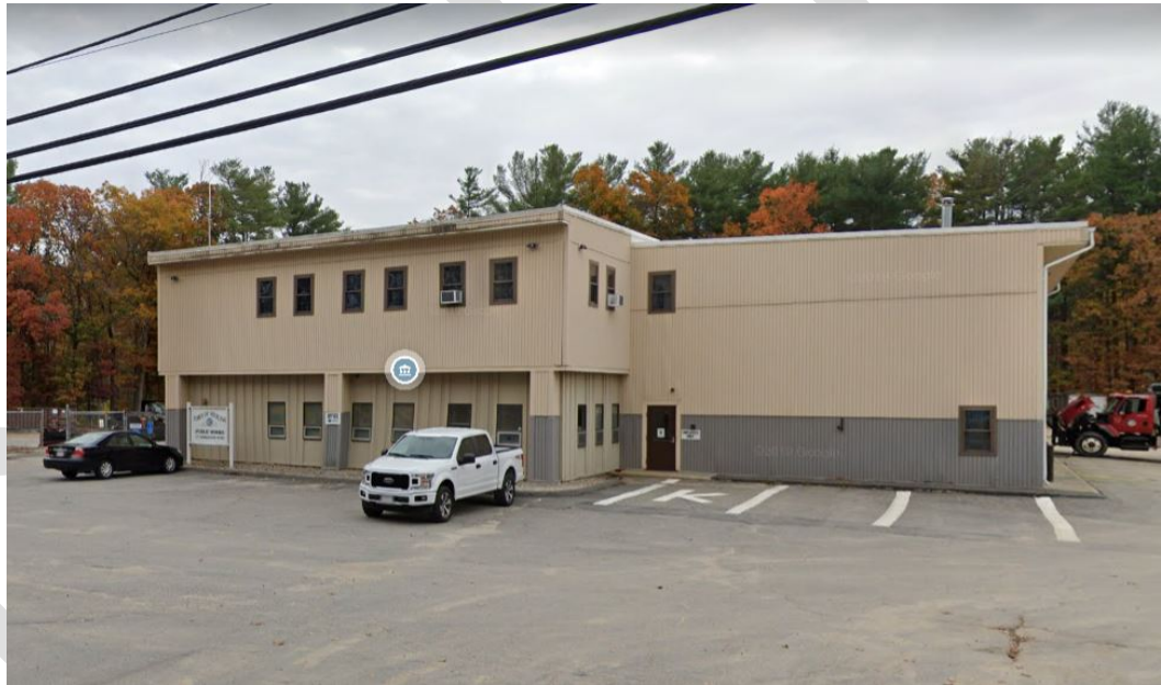
DPW Facility located at 171 Worcester Rd
