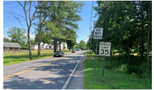
Image 5: Speed limit sign on Route 140 (Redemption Rock Trail) southbound that does not meet minimum sign height requirement (Site Visit July 2022)
